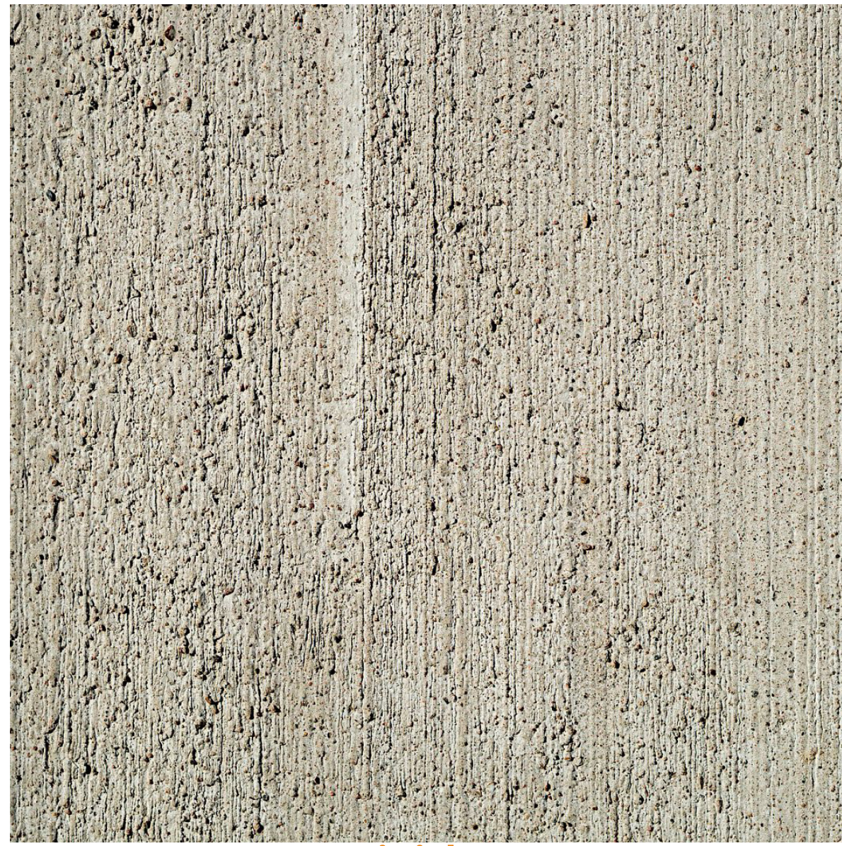
Concrete - Broom Finish
